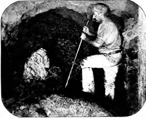
9.—De Beers Mine.—Underground Workings.
